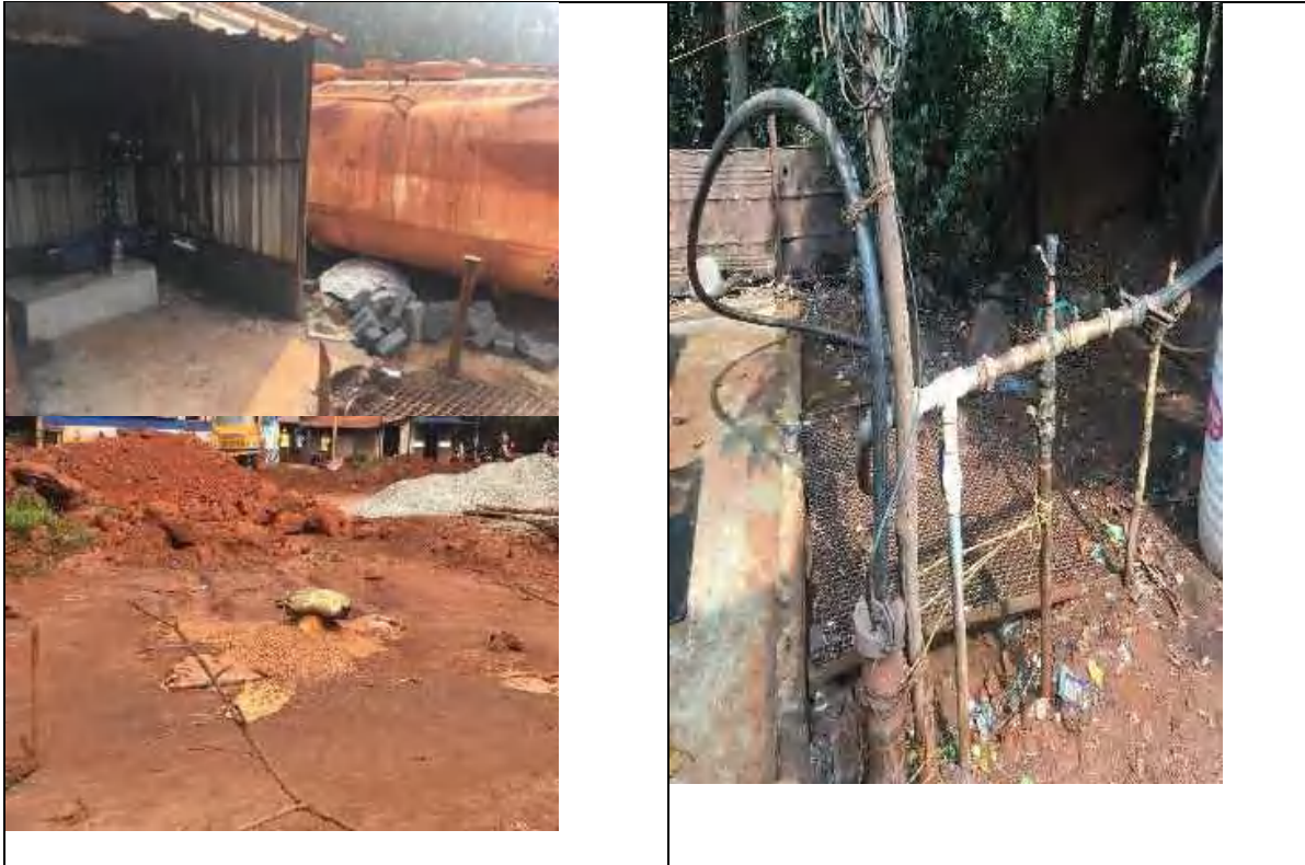
Picture 1: Photos of Bore well
