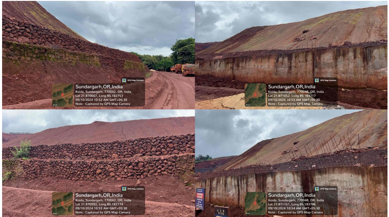
(View of Retaining wall around OB Dump)
